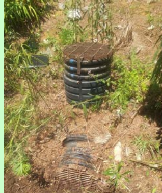
Outlet pipes with debris cleared off, but sediment still clogging the lower pipe which has since been removed
