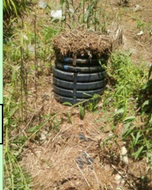
Outlet pipes clogged with debris after storm
