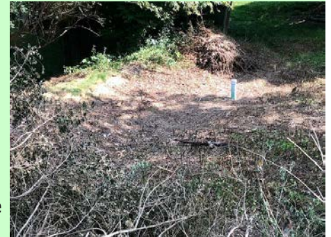
Cleared bio-detention pond with pile of brush
