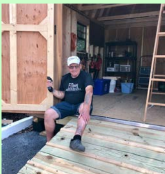
George Lally building a ramp for the shed
