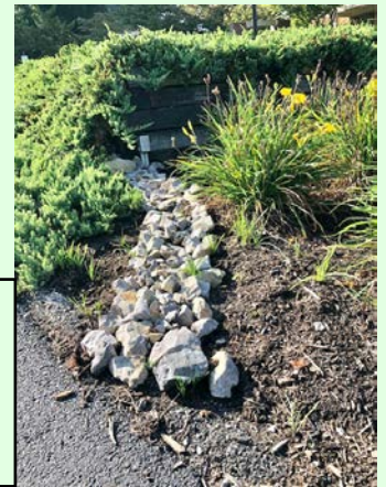
An erosion control measure to slow water flow from one of the parking lots and to keep mulch in place
