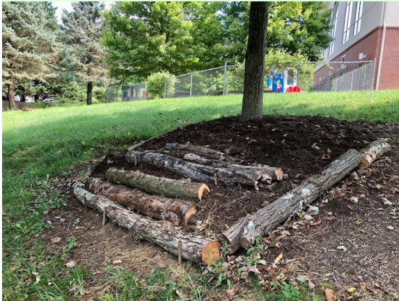
An erosion control measure to hold mulch in place on a slope
